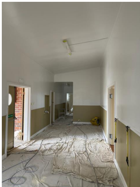
Railway Hall – Mould removal and painting (completed)
