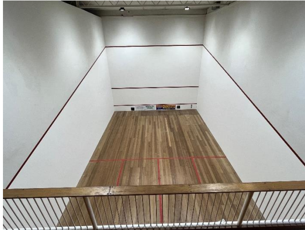
Wynyard Squash Centre – Painting Court Walls (completed)
