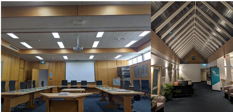
Wynyard Council Chambers and Atrium – LED Lighting Replacement (completed)
