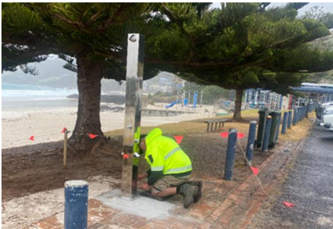
Installation of new outdoor shower at Boat Harbour Beach:
