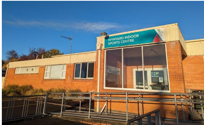
Window Replacement – Wynyard Indoor Sports Centre
