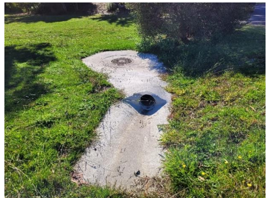
Figures 5 & 6 – Open drain clearing at Somerset and new Stormwater pit and entry at Stockdale Ave., Sister Beach
