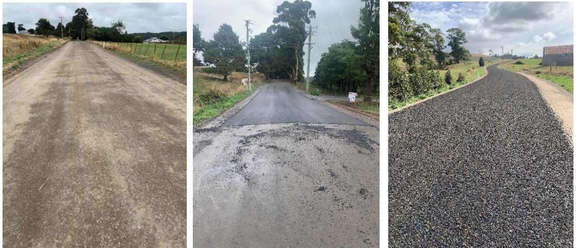
Figure 17, 18 & 19 – Sealing of Robin Hill Road, Flowerdale
