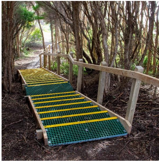
North-Western Stair replacement from Freestone Carpark to Bluff
