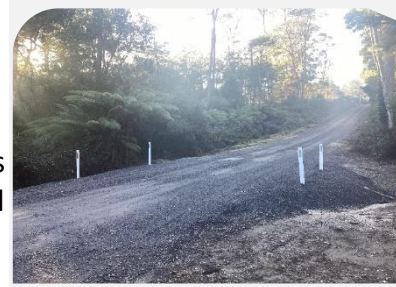
Ingleford Road Pipe Upgrade
