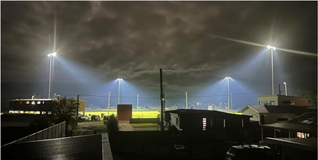
Langley Park Sports Lighting Upgrades (complete) – An action out of the Somerset Sports Precinct Master Plan
