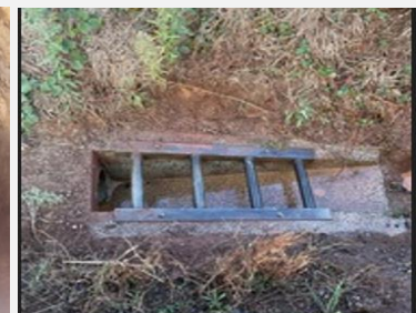
After - high-pressure water jetting
