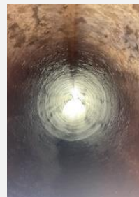
After - high-pressure water jetting
