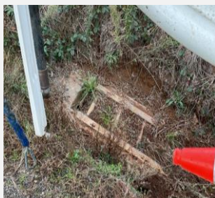
Before - high-pressure water jetting
