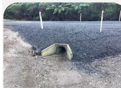
Ingleford Road Pipe Upgrade
