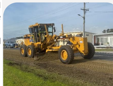
Old Bass Highway Shoulder Grading
