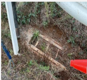
Before - high-pressure water jetting
