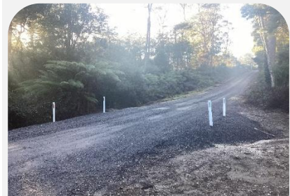
Ingleford Road Pipe Upgrade
