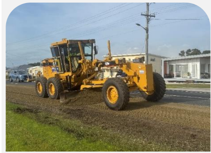
Old Bass Highway Shoulder Grading
