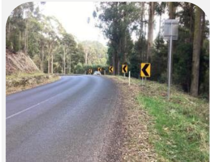
Rural Road Safety Audit Signage
