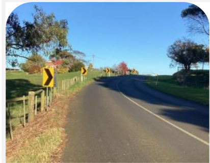
Rural Road Safety Audit Signage
