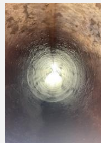
After - high-pressure water jetting
