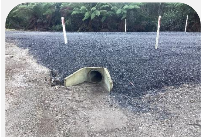
Ingleford Road Pipe Upgrade
