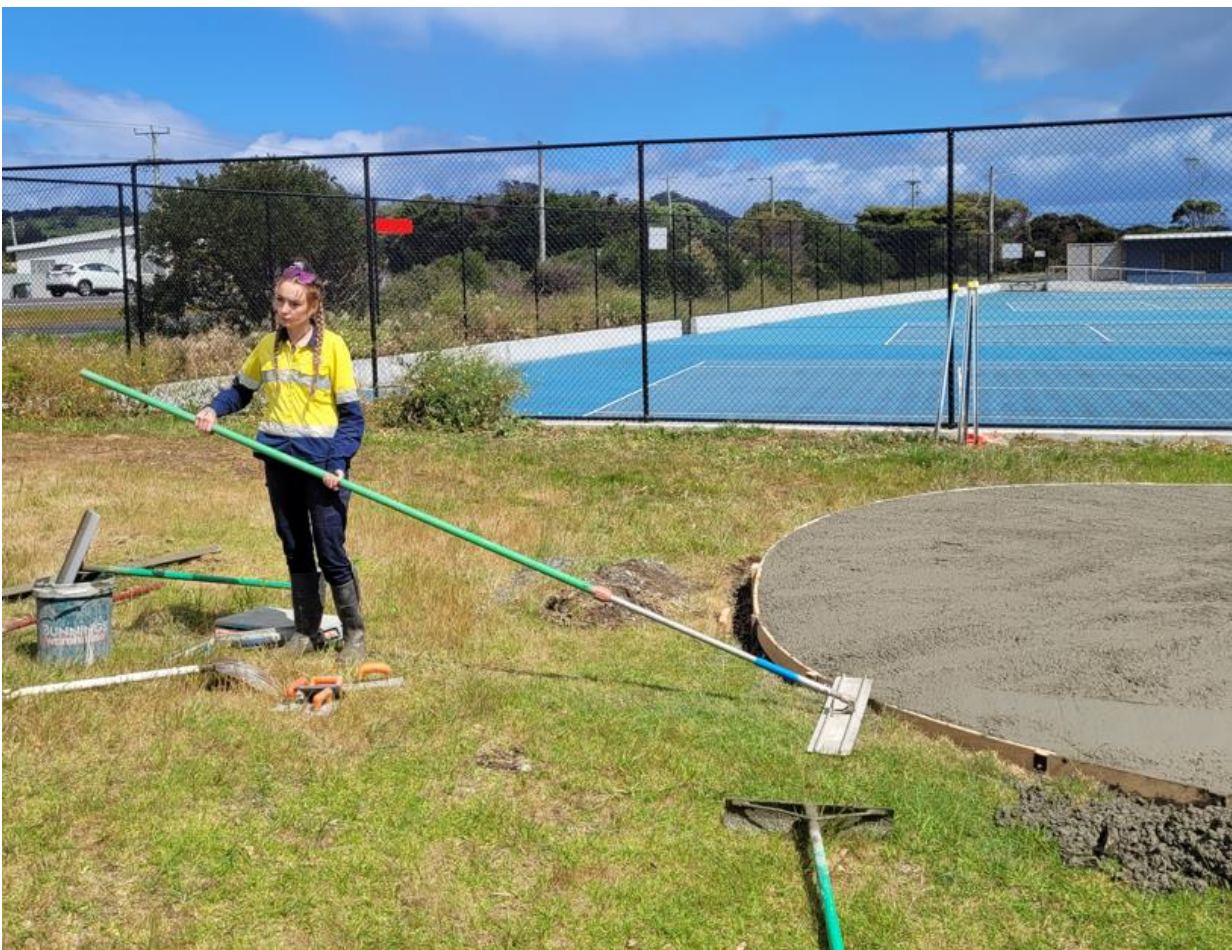
Civil trainee pouring a new concrete slab, adjacent the Coastal Pathway in Somerset
