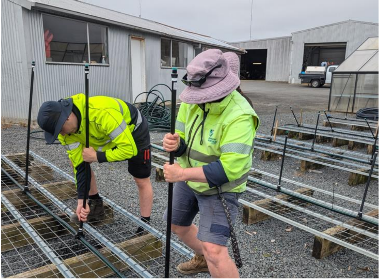
Athol St driveway repairs
