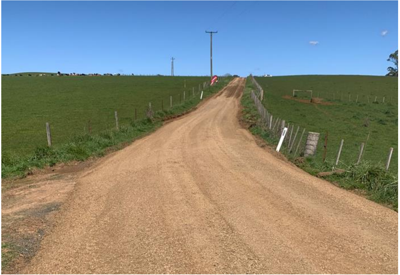
Shoulder grading of Mt Hicks Rd
