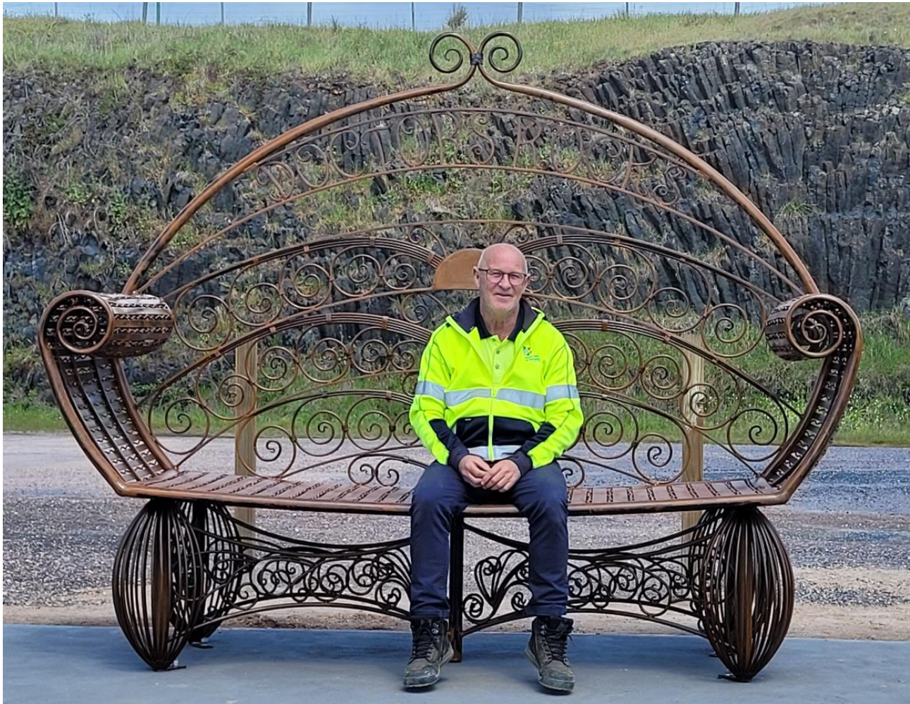
River track storm repairs
