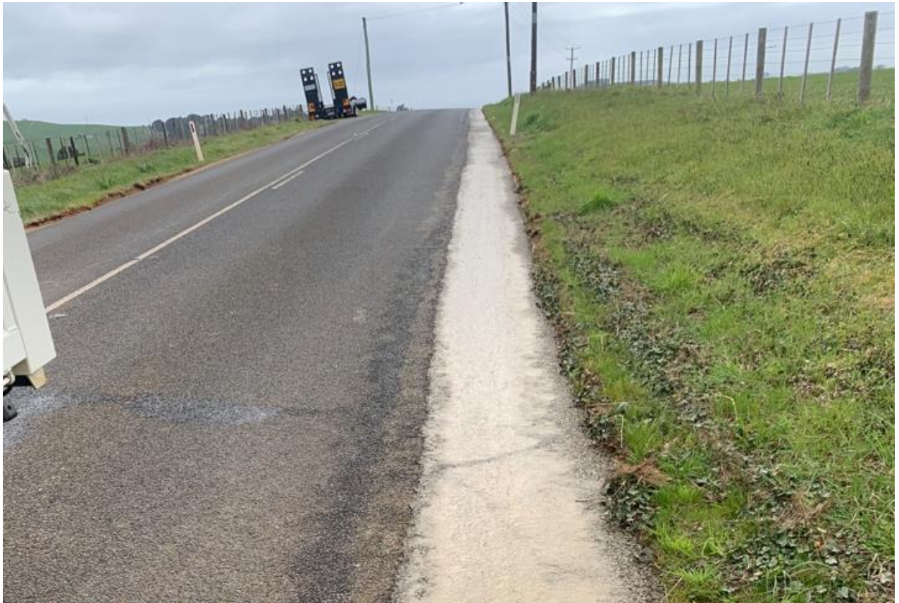
Shoulder grading of Mt Hicks Rd
