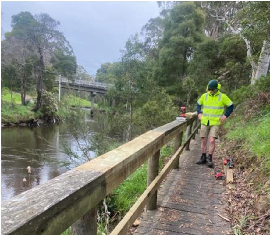
Re-sheeting of Aitkins Rd
