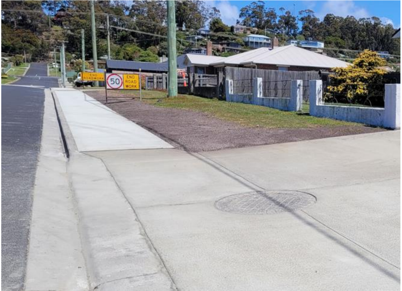
Wynyard Rec. asphalting
