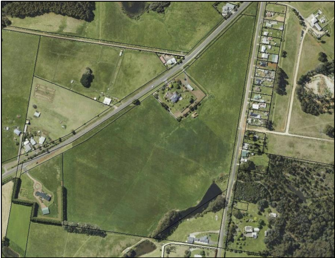
Figure 2: Aerial image of site and surrounds (Source: ListMap)
