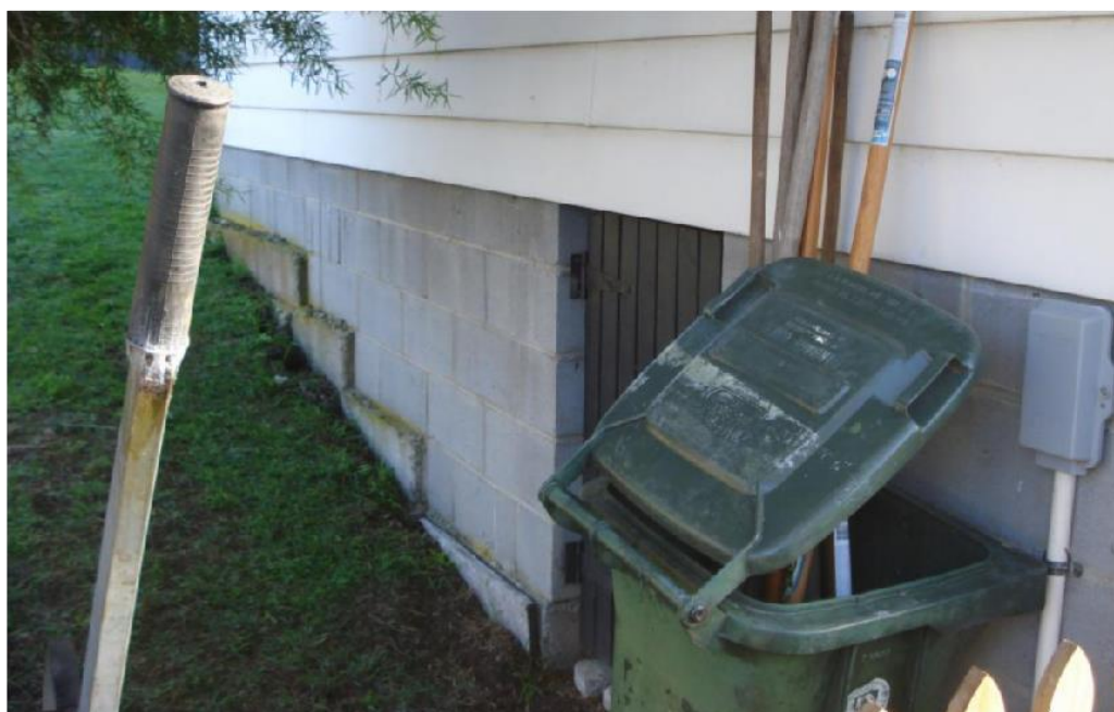
Photo 2. Exposed parts of existing footings, test pit was excavated along this wall
