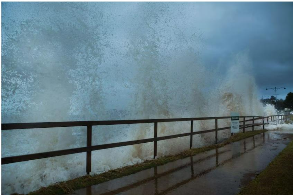
King tides coupled with a storm surge smashed the Penguin foreshore in the winter of 2018. (ABC Northern Tasmania: Rick Eaves)
