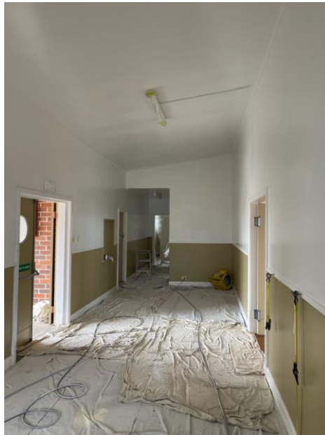
Railway Hall – Mould removal and painting (completed)
