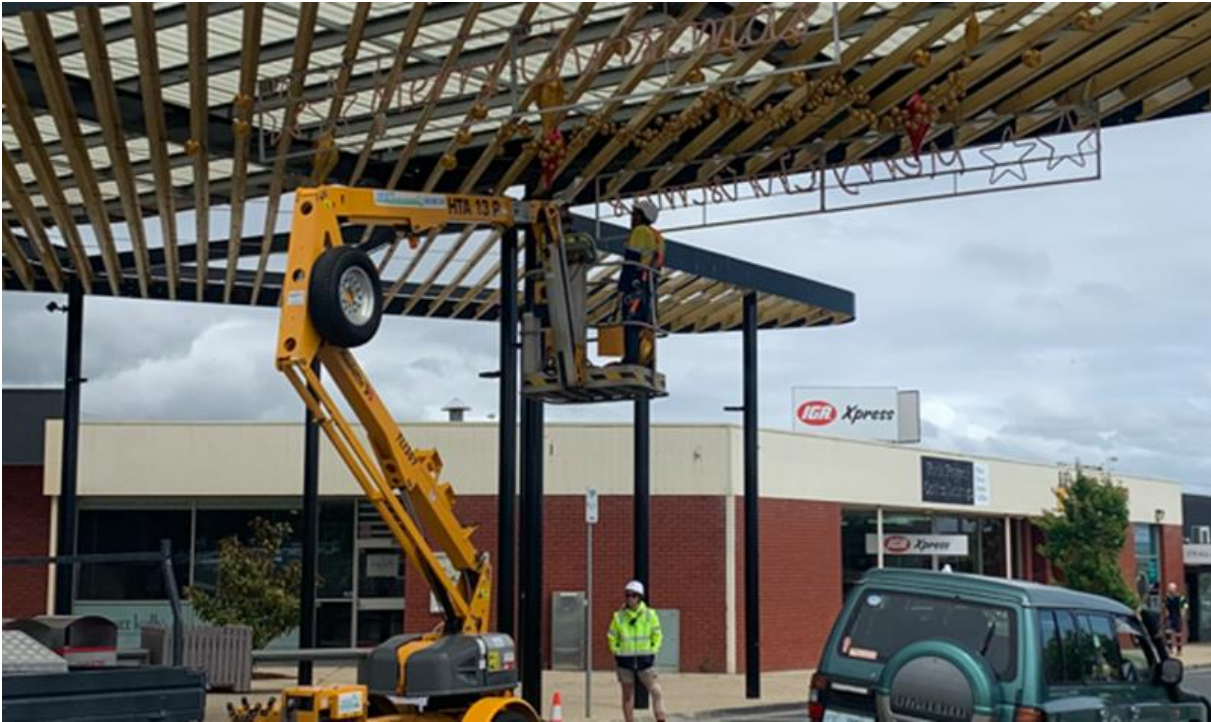
Installation of Christmas Decorations at the Somerset Plaza:
