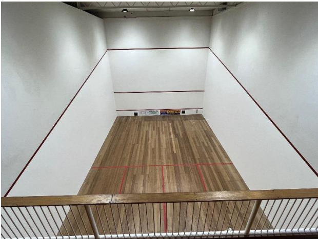
Wynyard Squash Centre – Painting Court Walls (completed)
