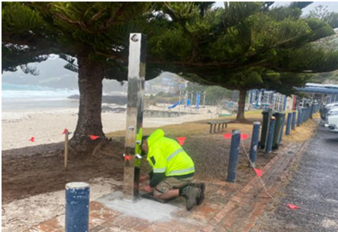
Installation of new outdoor shower at Boat Harbour Beach:
