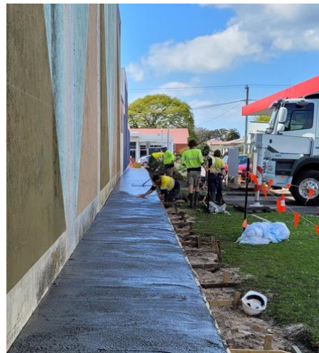
Figure 17 & 18 – Dares Rd, Myalla resheeting and a big concrete pour for the footpath at Jackson St
