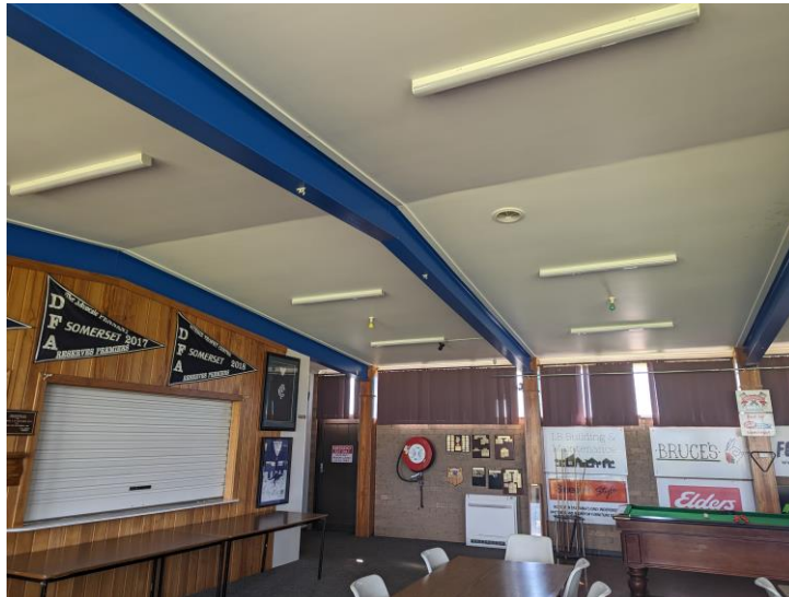
Langley Park – LED lighting replacement
