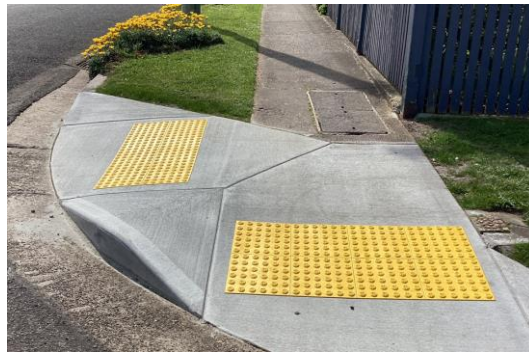
Figures 23 & 24 – Resheeting on Smart Hills Road and TGSIs installed on Saunders St footpath kerb ramps
