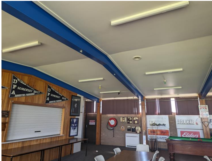
Langley Park – LED lighting replacement
