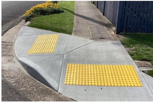
Figures 23 & 24 – Resheeting on Smart Hills Road and TGS’s installed on Saunders St footpath kerb ramps
