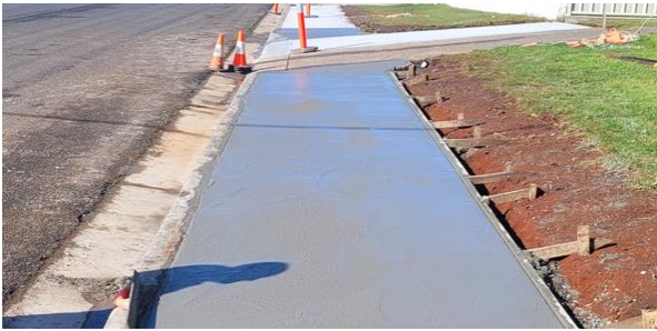
Figures 9 & 10 - 2nd pour for Hogg St footpath and shoulder grading on Lapionya Rd
