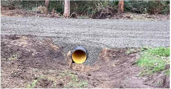
Figures 11 & 12 – New culvert installed on the Inglis River Walking Track and Wicket renovations at Wynyard Rec Grounds
