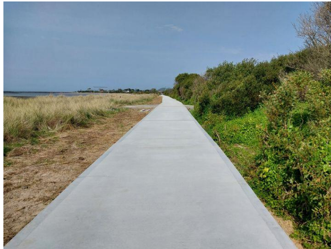
East Wynyard Foreshore – Walking track completion (replacement of boardwalk)
