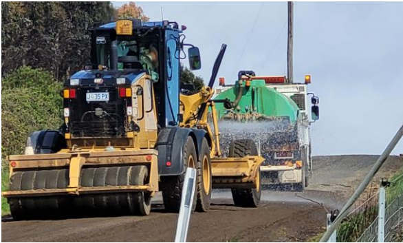
Figures 23 & 24 – Resheeting on Smart Hills Road and TGS’s installed on Saunders St footpath kerb ramps
