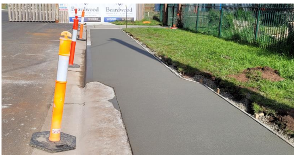
Figures 7 & 8 - Hogg St footpath – 1st pour completed and made over garden bed at Inglisdale Drive
