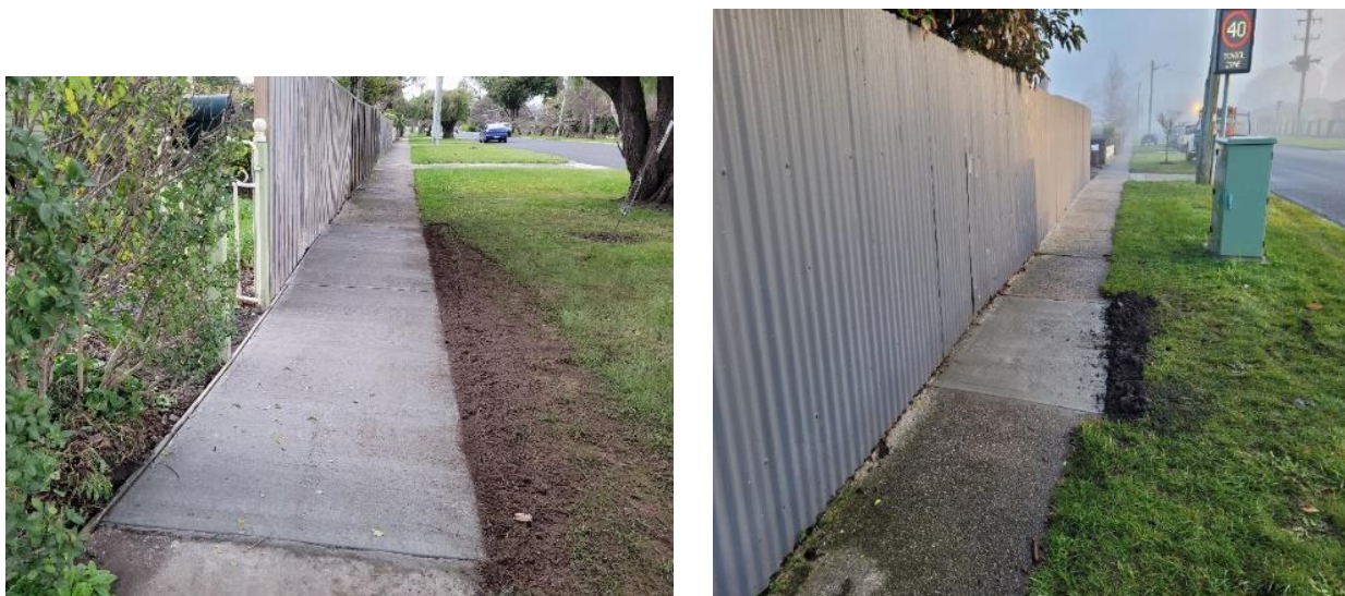
Figures 12 & 13 – Footpath repaired section on Saunders Street and Church Street
