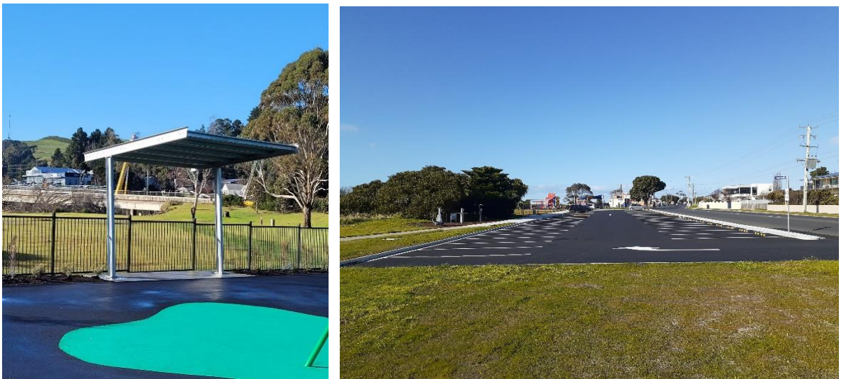
Figures 29 & 30 – One off the three new shelters at Anzac Park and the now finished East Wynyard Car Park
