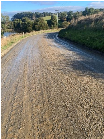
Figure 17, 18 & 19 – Corrugated gravel road corner improvements on Gates, West Calder and Scotts Roads
