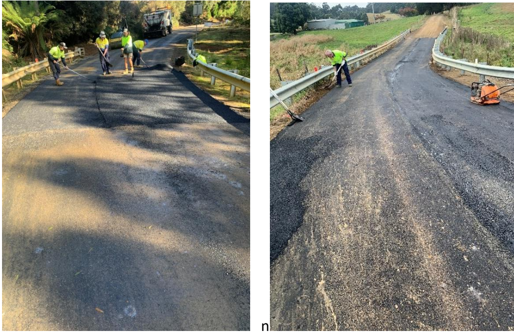
Figure 28 – Bridge approach sealing Takone and Coates Roads
