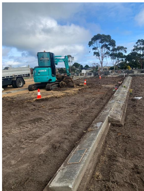
Figures 5 & 6 – Turf Bar Lowering at Wynyard Cemetery
