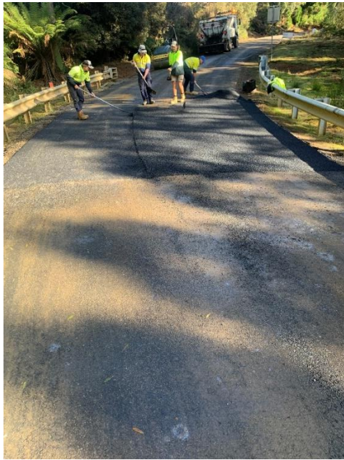
Figure 28 – Bridge approach sealing Takone and Coates Roads
