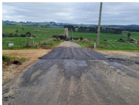
Figures 7, 8 & 9 – Tysons Rd culvert and verge maintenance, typical tree limb hanging that requires attention and section of hot mix replacement over damaged cattle crossing on Nunns Road
