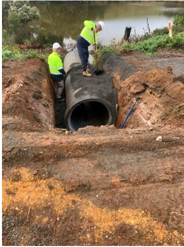
Figures 26 & 27 – Installation of new culvert on Gates Road
