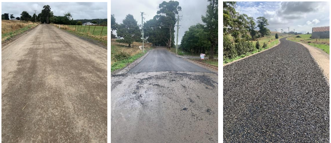
Figure 17, 18 & 19 – Sealing of Robin Hill Road, Flowerdale
