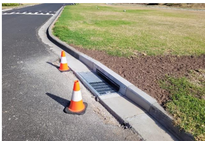
Figures 1 & 2 Culver clearing on Calder Road and a new Side Entry Pit on the Esplanade in Somerset
