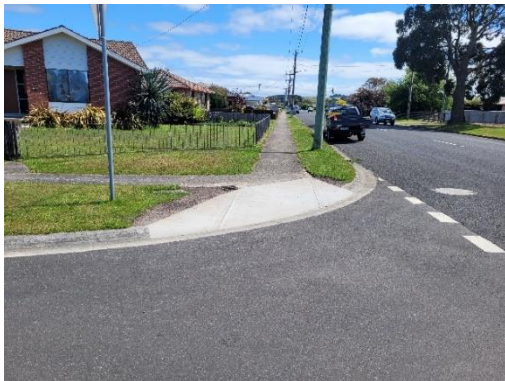
Figures 16, 17, 18 & 19 – New DDA Ramps at Simpson St., Stanwyn Crt., Inglis St. and Lewis/Beauford St.
