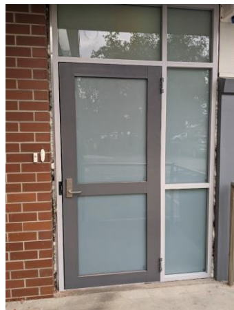
Upgraded doorway – Council Chambers
