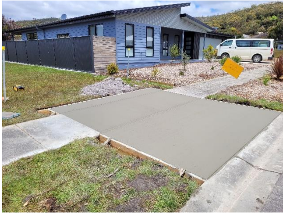
Figure 20 – New driveway at Serrata Crescent
