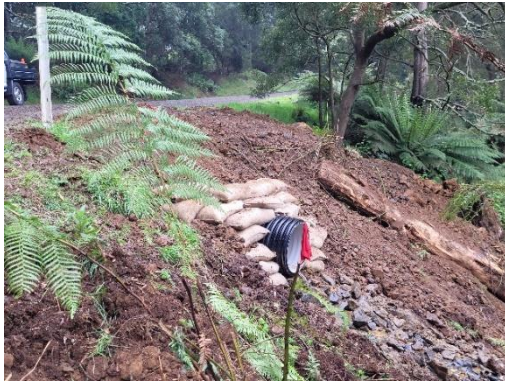
Figures 21 & 22 – Installation of new culverts at South Elliot Rd. and Zig Zag Rd.
