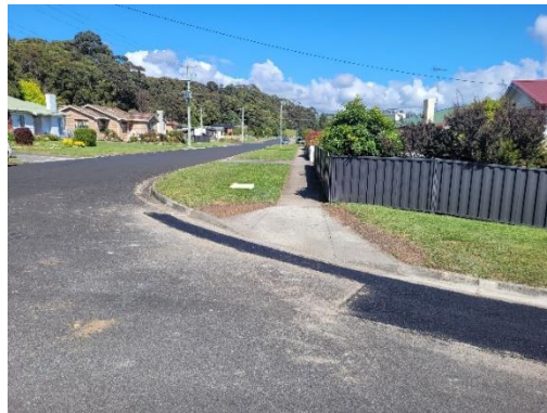
Figures 16, 17, 18 & 19 – New DDA Ramps at Simpson St., Stanwyn Crt., Inglis St. and Lewis/Beauford St.
