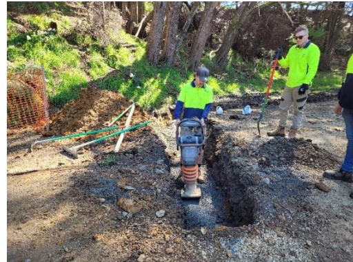
Figures 21 & 22 – Installation of new culverts at South Elliot Rd. and Zig Zag Rd.
