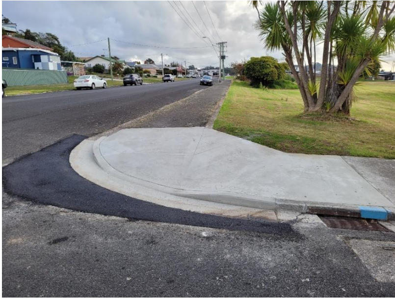
DDA footpath ramps in Somerset
