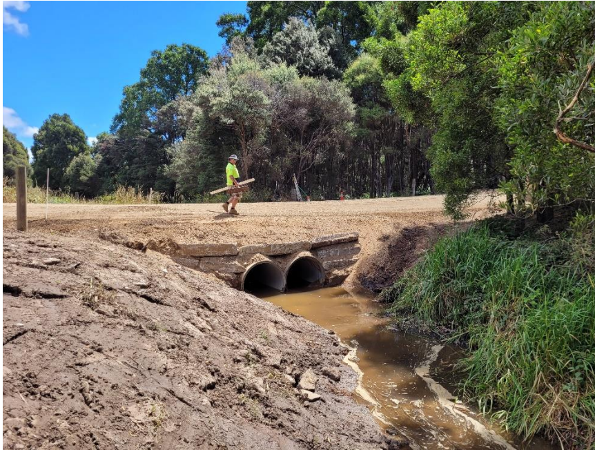
New culvert and road widening at Blackabys Road.
