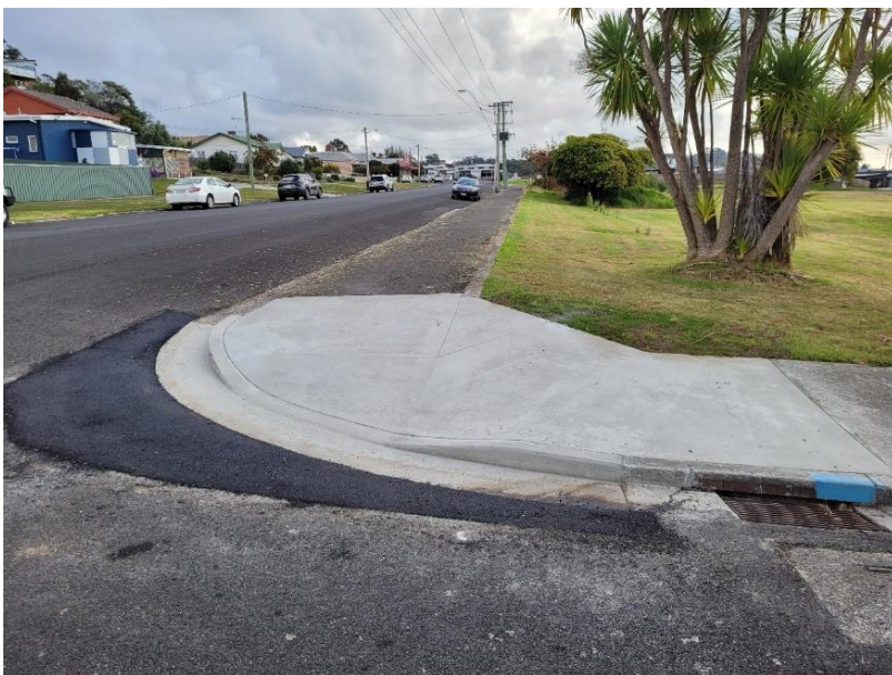
DDA footpath ramps in Somerset
