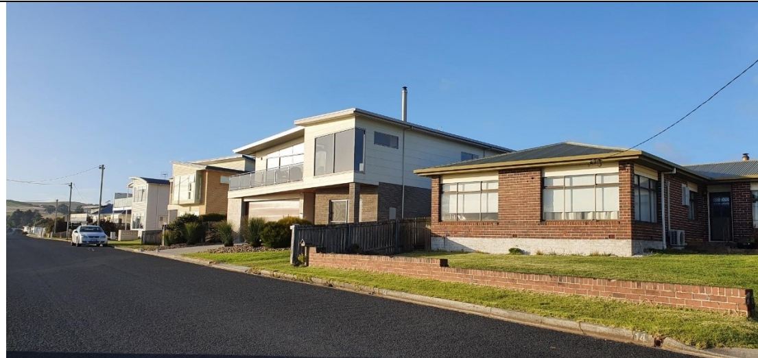
Figure 4 - Streetscape of subject site looking towards 14a Somerset Esplanade.
