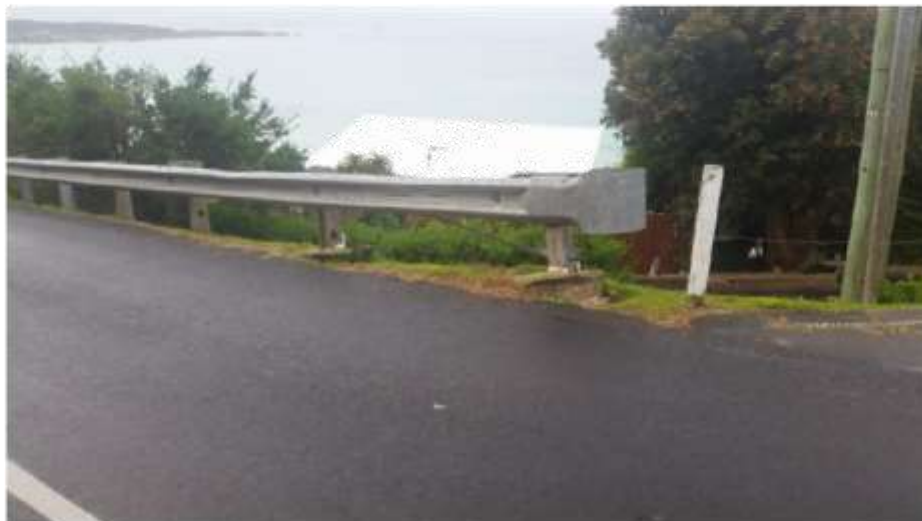
Photo 2. Guard posts along Port Road being pulled out of the ground.
