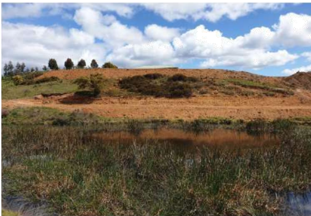
Photograph looking west from the opposite side of the waterway towards the earthworks. Notably, there is a band in the middle where existing grass and vegetation is maintaining slope stability. Some minor landslide present.
