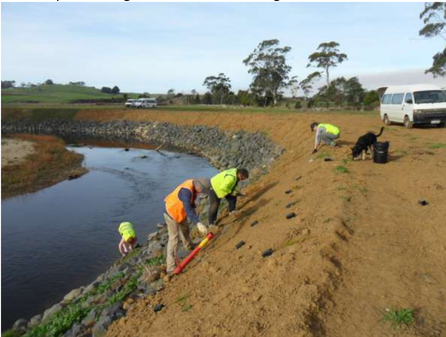
An example of revegetation works occurring.
