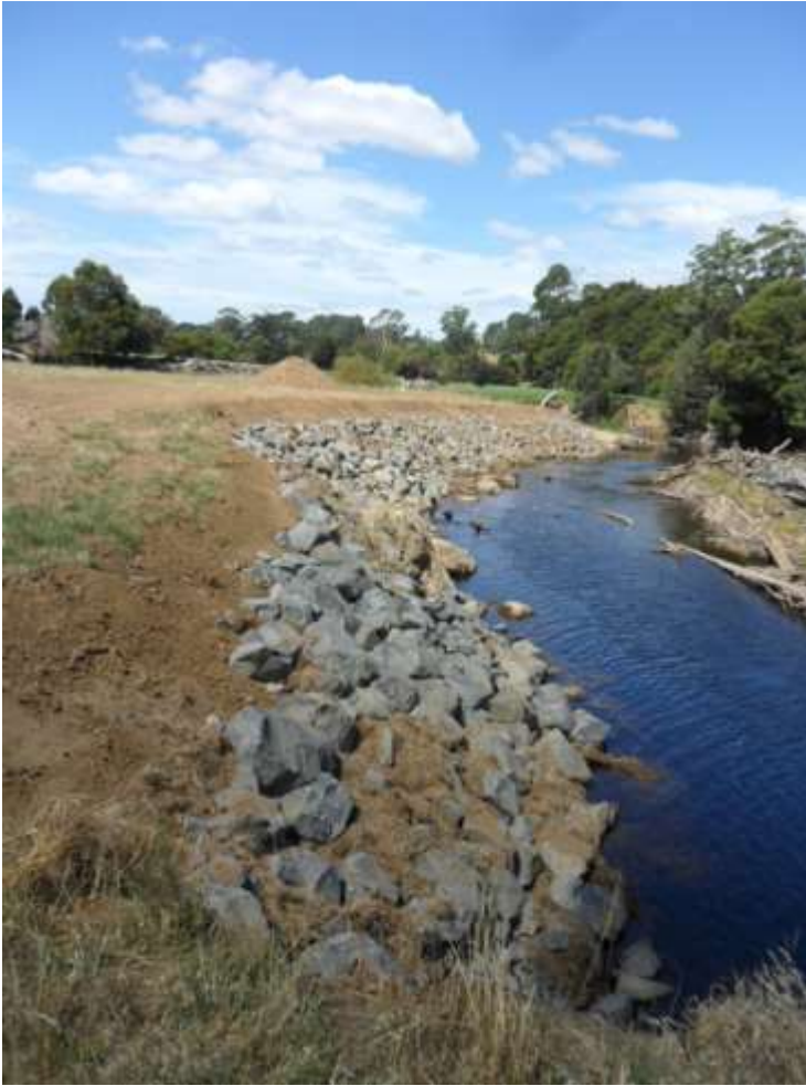
After rock armouring completed
