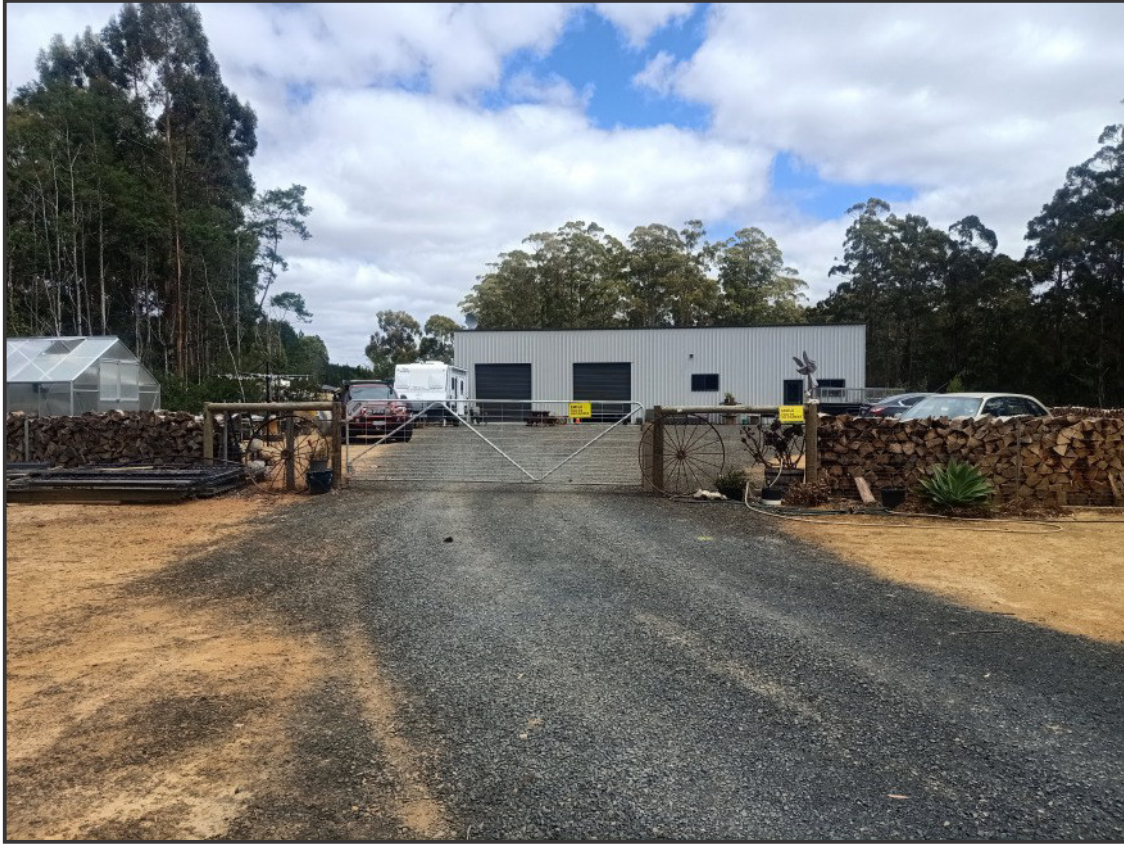
PLATE 1 - View of the existing shed looking to the west
