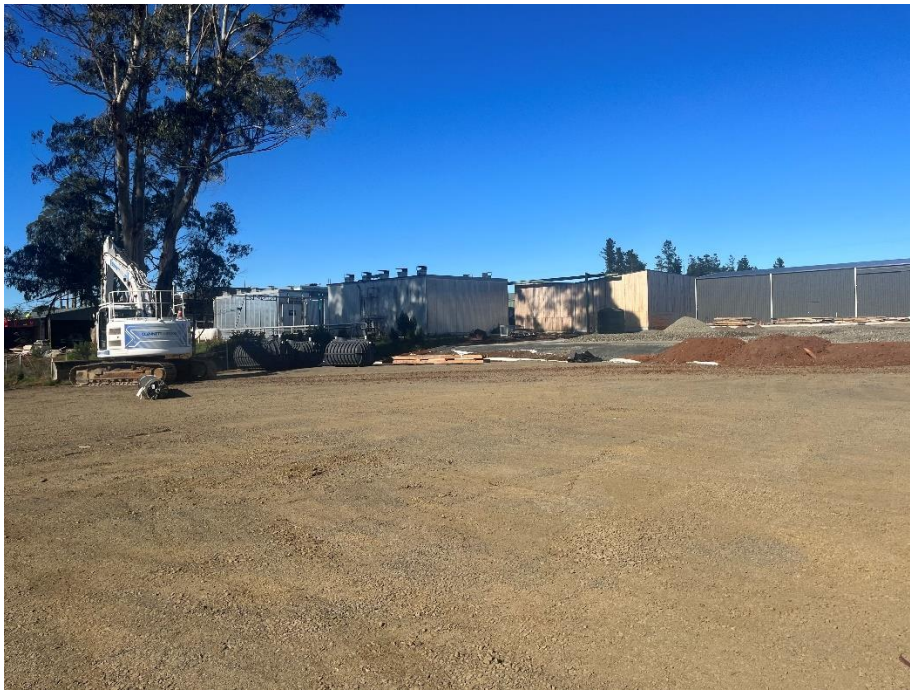
Image 4.1.2 – South - low threat existing sheds and accesses
