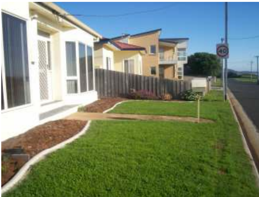
Figure 2 – View across adjoining landowner situated on the north-eastern boundary. The subject building is shown with a red roofline (second from front).
